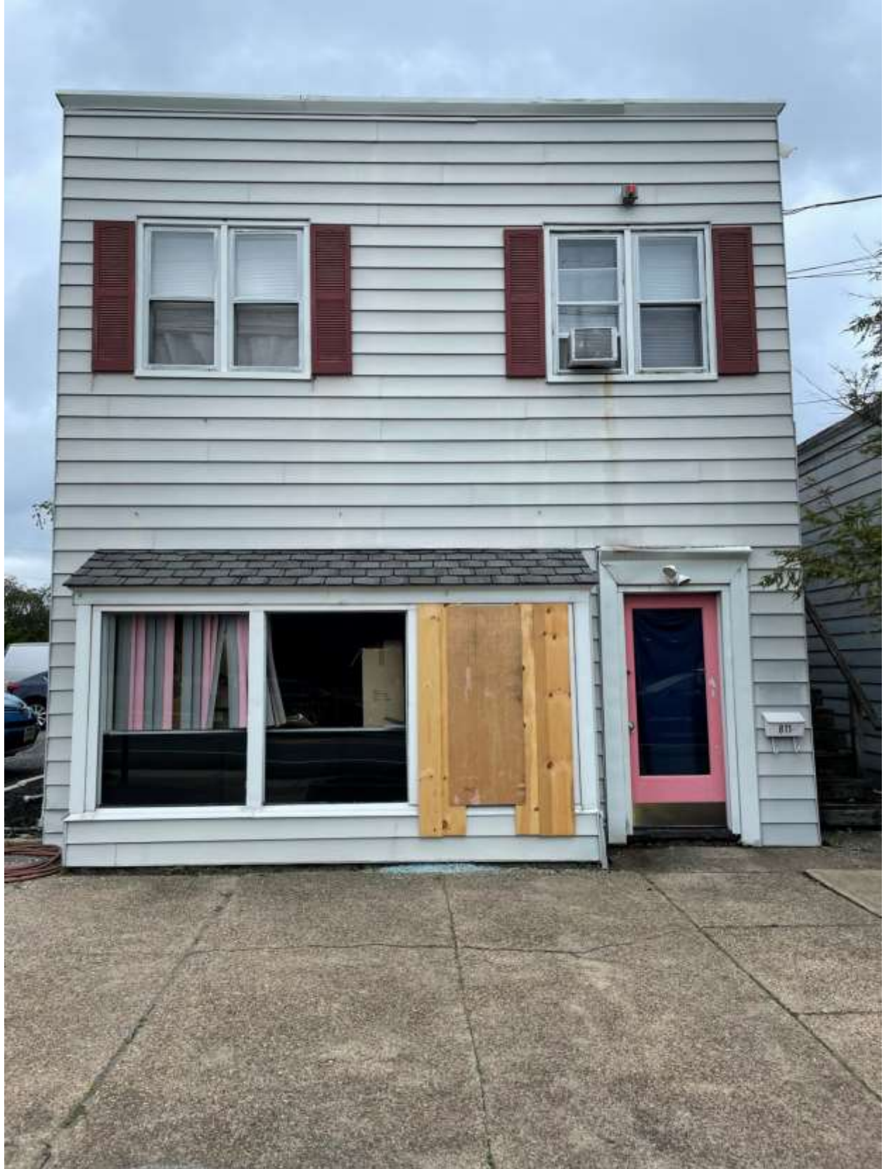
2Existing Building Facade
